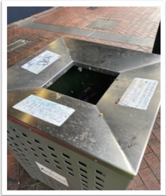
Image 5 - Bin enclosure - 64 Gouger Street - before
