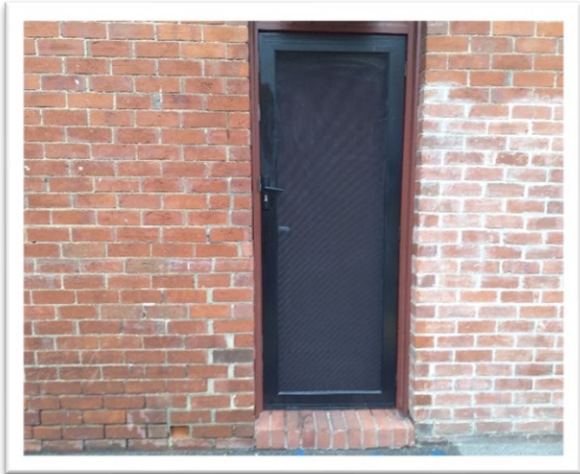
Image 10 - Graffiti removed from side door – after
