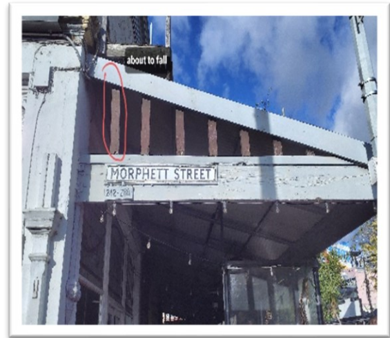
Image 22 - Loose railing.
