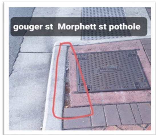
Image 1 - Gap between pit surround and kerb at the intersection of Gouger Street and Morphett Street
