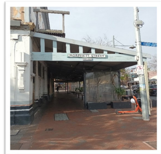
Image 23 - Loose railing fixed.
