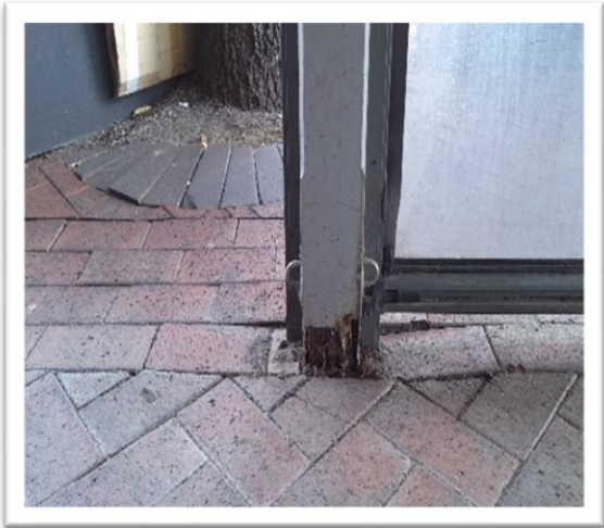
Image 24 - Damaged footing
