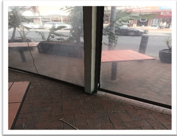
Image 25 - Damaged footing fixed
