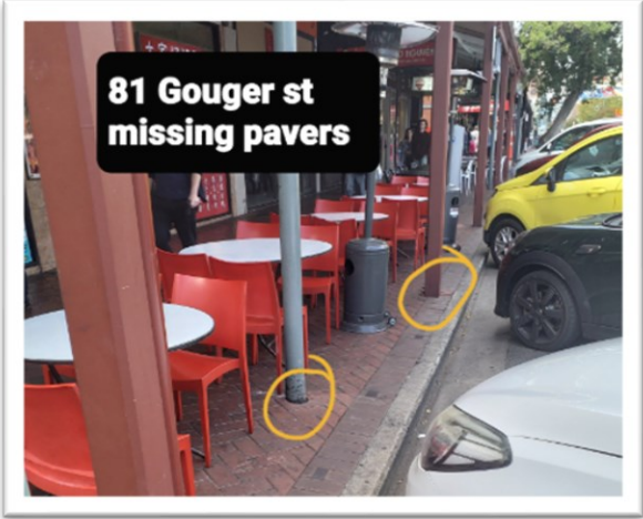
Image 5 - Missing pavers and gaps noted at base of veranda poles at 81 Gouger Street
