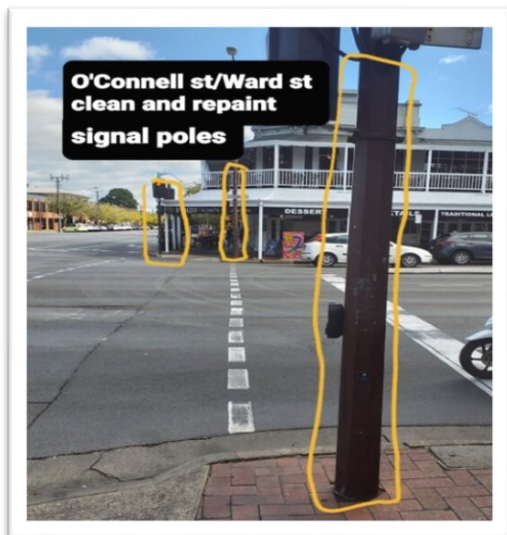
Image 49 – Poles identified through collaborative action.
