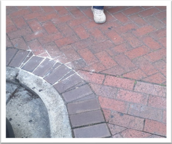
Image 4 - Loose pavers repaired and sweeping sand applied.
