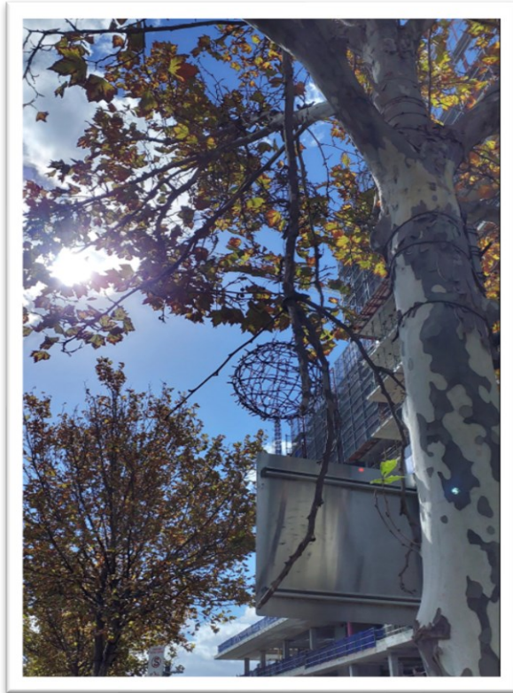
Image 42 - Branch requiring removal 88 O'Connell Street
