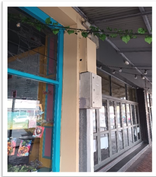
Image 21 - Fuse box cover fixed
