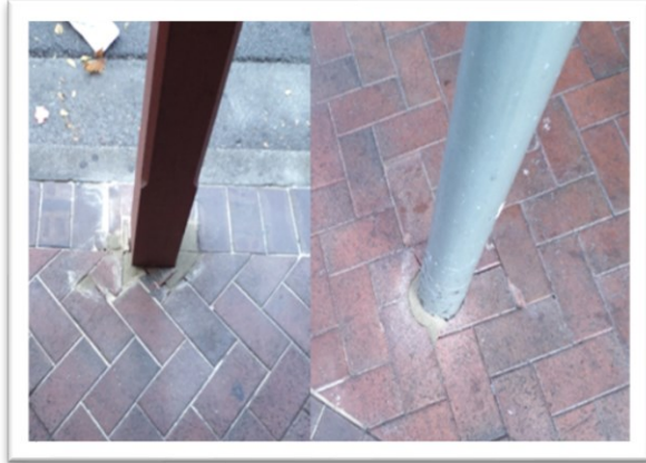
Image 6 - Pavelock and pavers placed at base of veranda poles.
